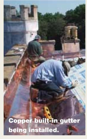
Copper built-in gutter being installed.
