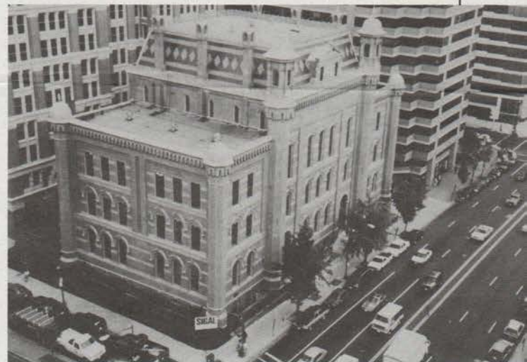
The Franklin School restoration, shown completed above, lasted almost a year.
